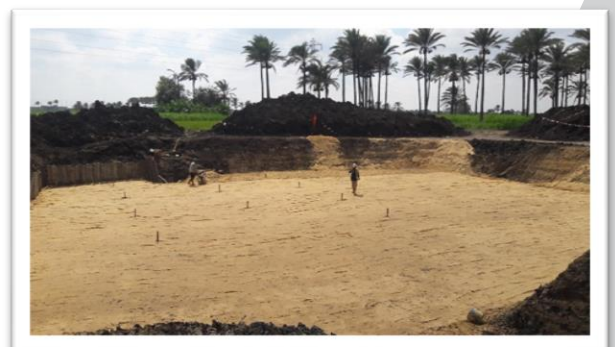
Soil replacement and compaction
