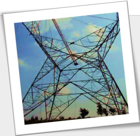
500 kV Single Circuit Tower
