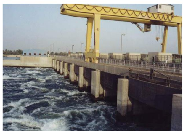
ESNA Hydro Power Plant
