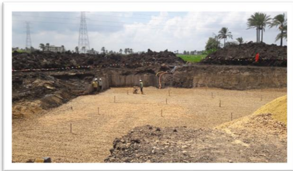
Soil replacement and compaction
