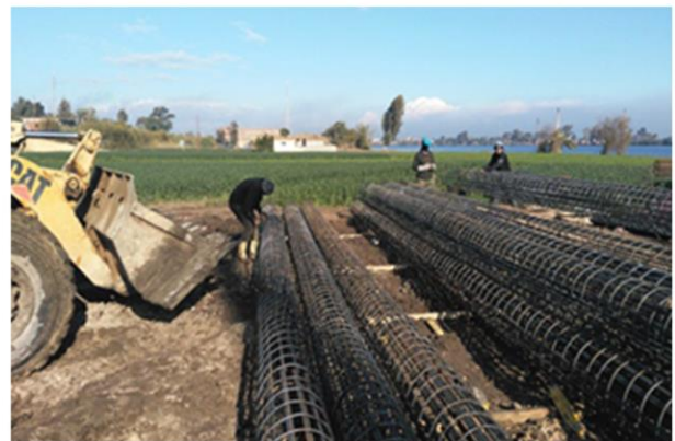
Deep Foundations (Piles) for OHTL
