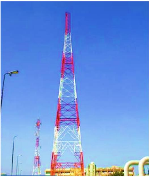
Design & Construction Supervision Of MicroWave Towers
