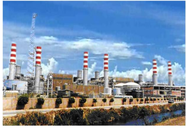
Damietta Combined Cycle Power Station
