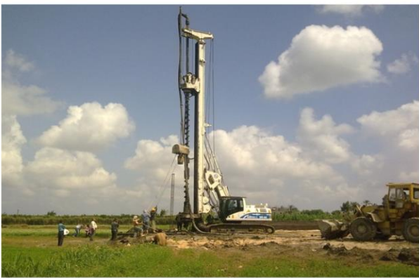
Deep Foundations (Piles) for OHTL
