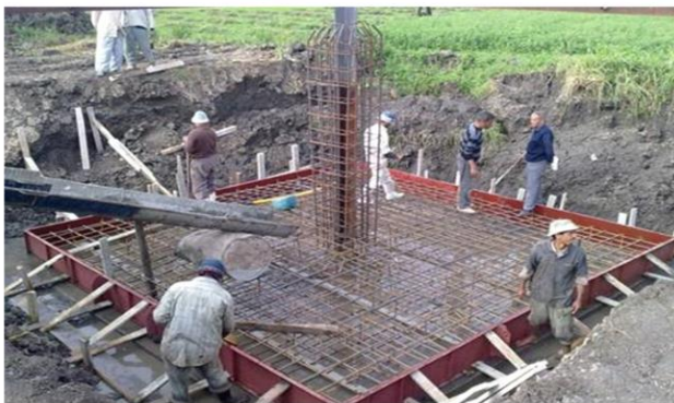
Foundation for OHTL
