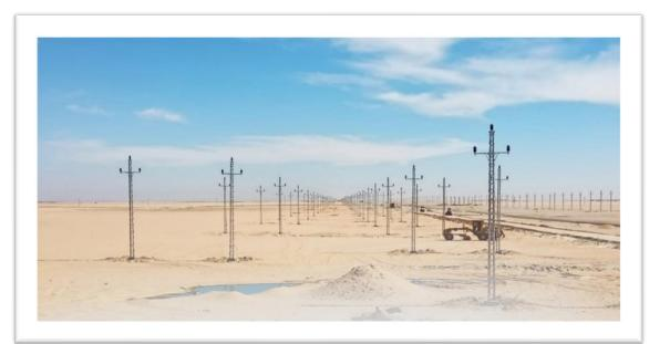
**OverHead Transmission Lines 22kV**
