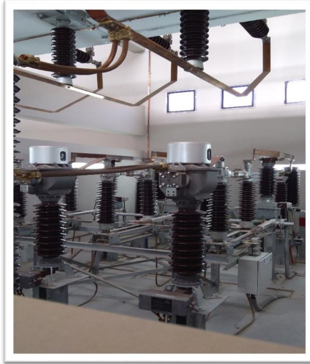
Conventional Indoor 66 kV Equipment
