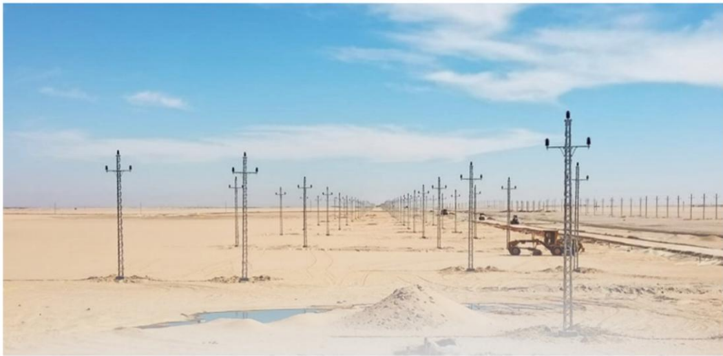
OverHead Transmission Lines 22kV
