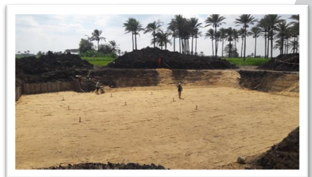
Soil replacement and compaction
