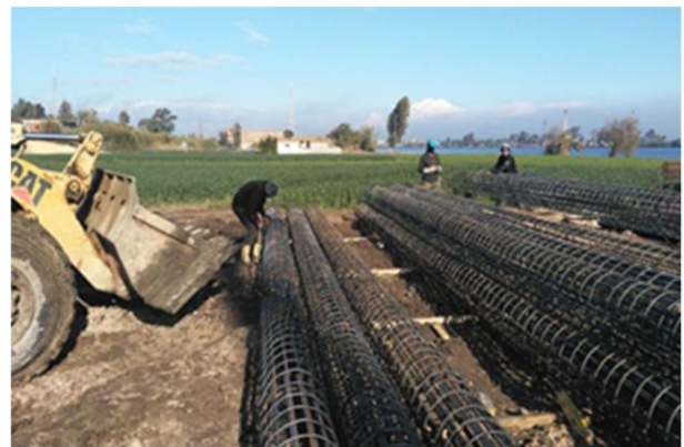
Deep Foundations (Piles) for OHTL
