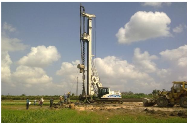
Deep Foundations (Piles) for OHTL
