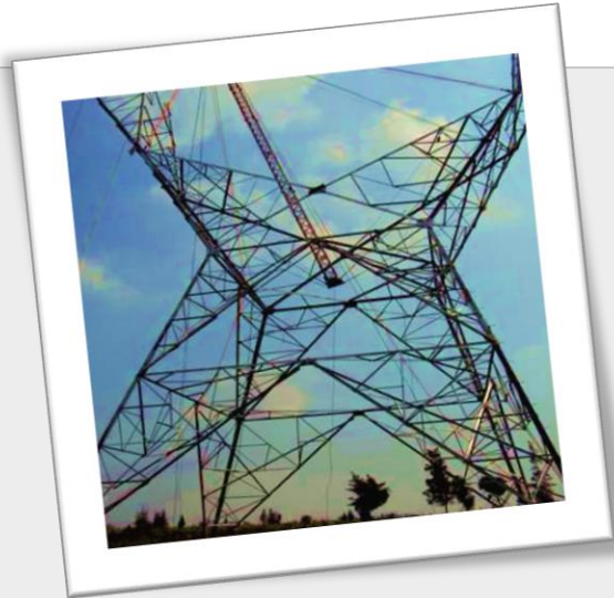
500 kV Single Circuit Tower
