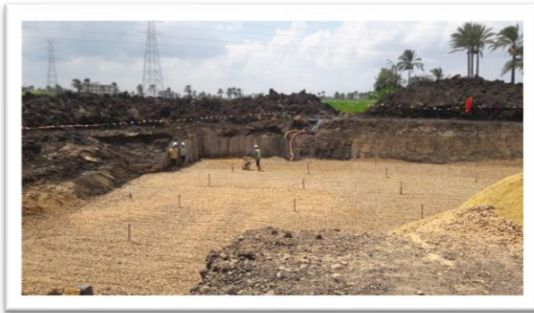
Soil replacement and compaction
