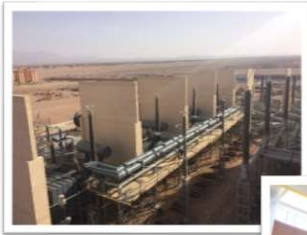
Suez Gulf 500/220 KV GIS Substation 1x500 MVA
