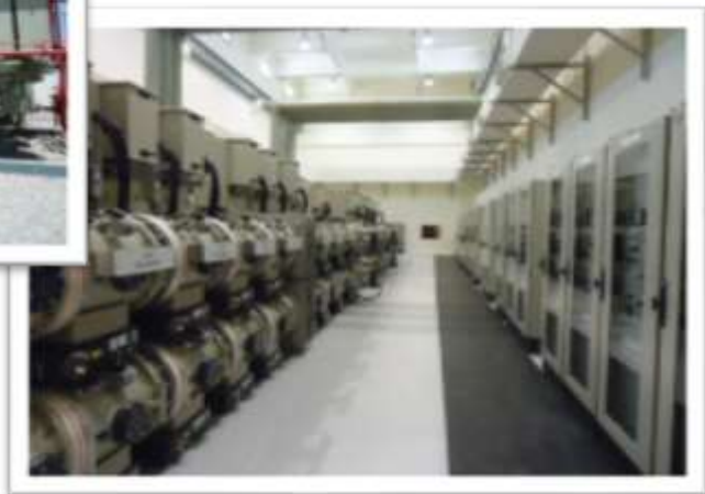
New Ghobrah 132/33/11 KV GIS S/St
