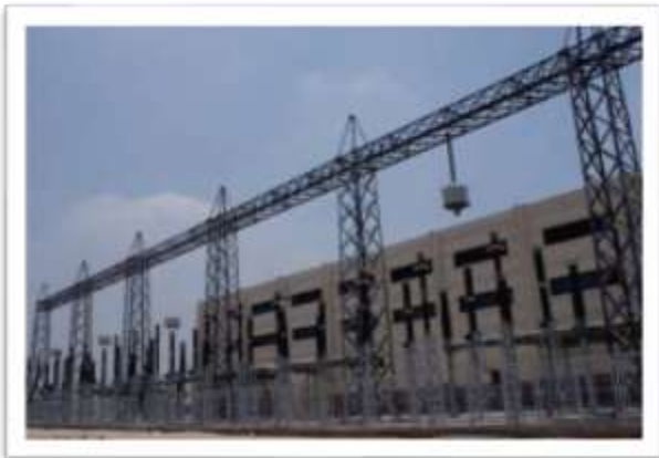
Kafr El Zayt 220 kV Outdoor Equipment
