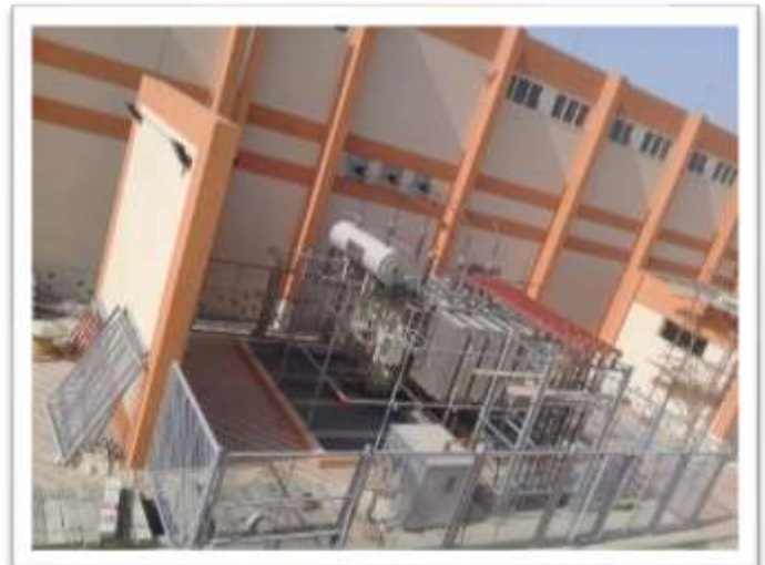
United 66/11 kV Substation
