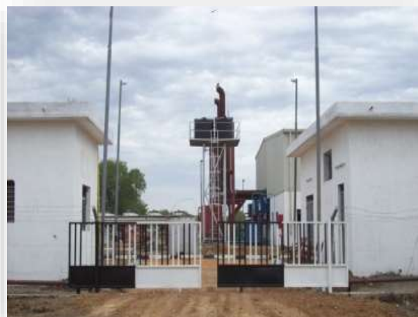
Bor Power Plant Main Entrance
