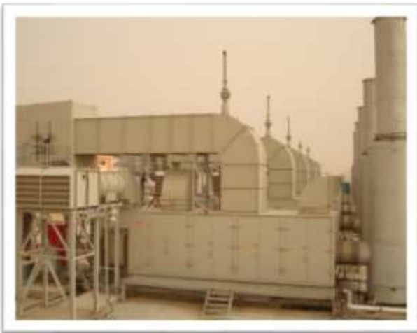
Karama Power Plant
