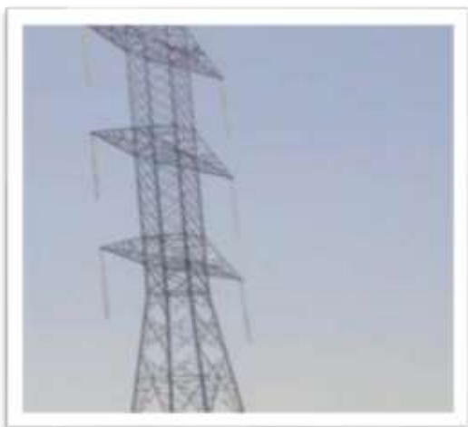
500 kV Double Circuit Tower
