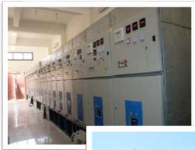
Medium voltage Switchgear
