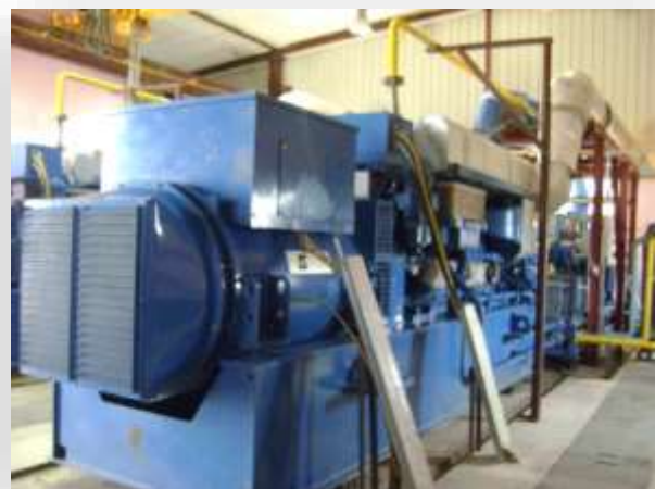
Diesel engines inside engine hall
