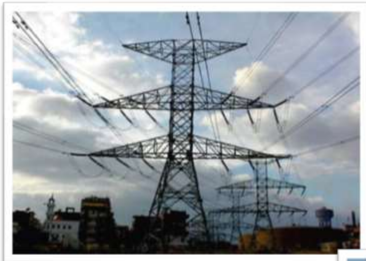
Multi Circuits Towers Approach to El-Siouf Substation
