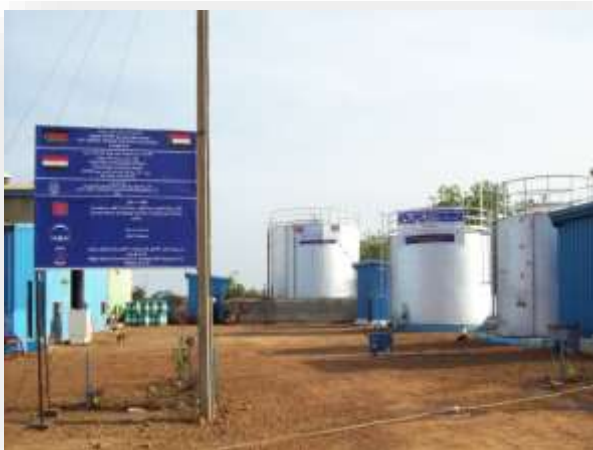
Wau Power plant over View
