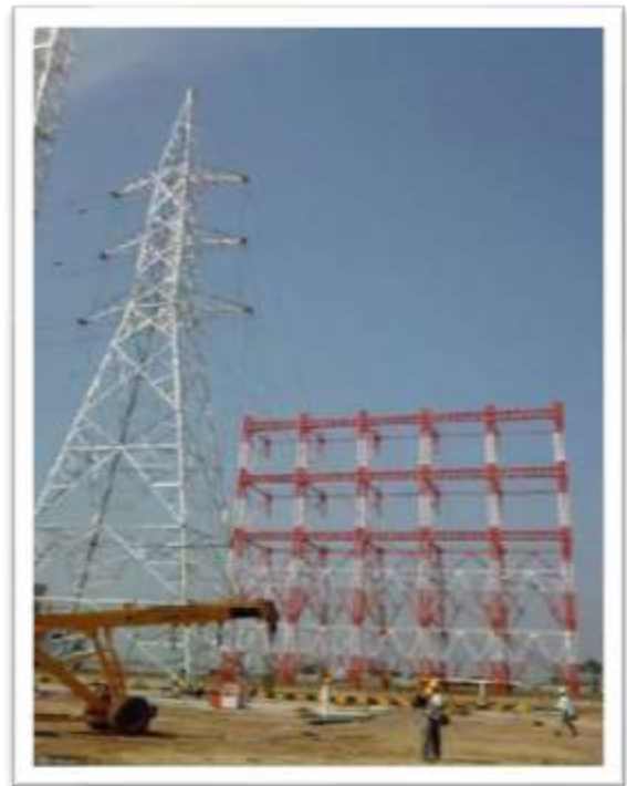
Loading test for Towers
