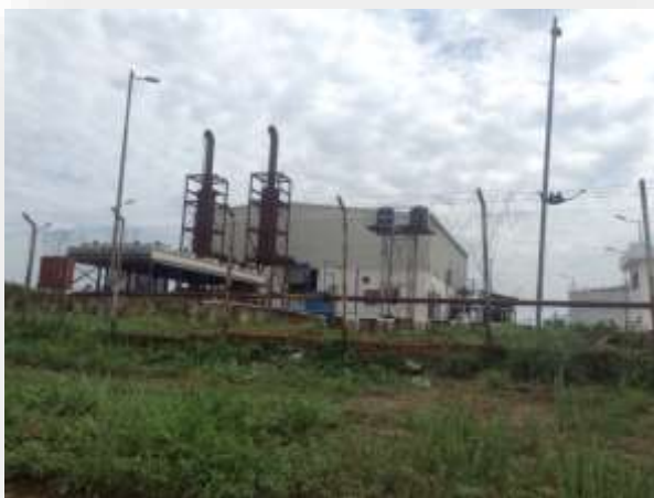
Yambio Power plant over View
