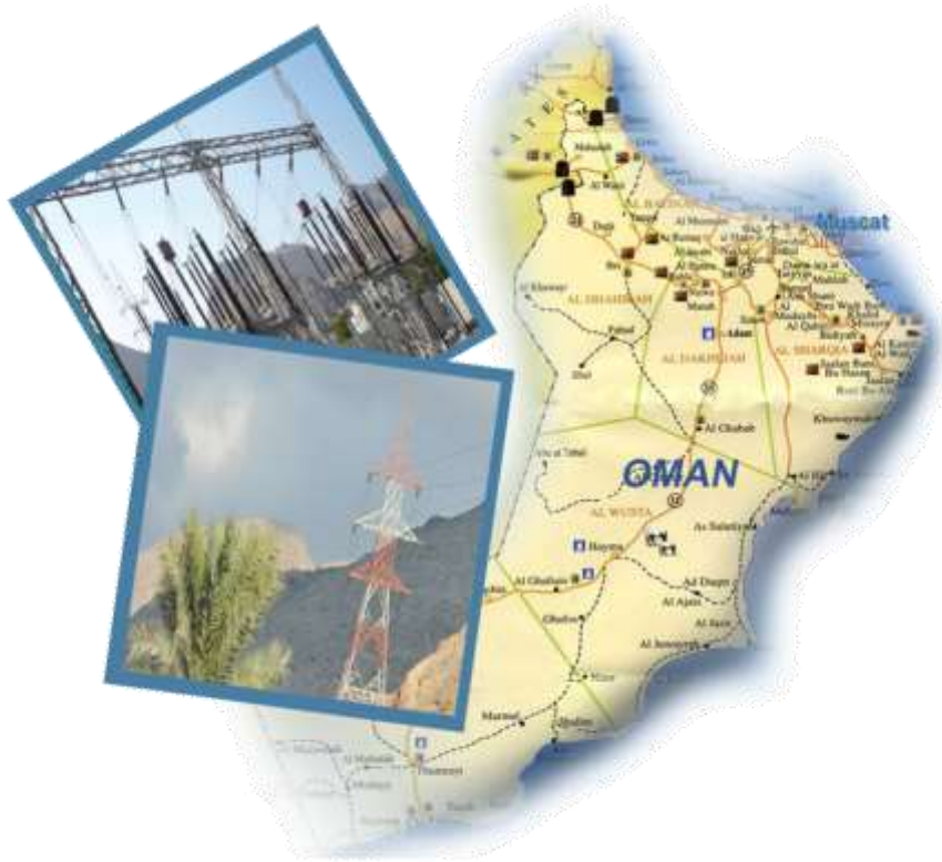
Substation & Transmission Line Oman
