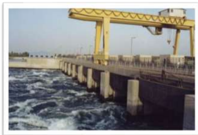
ESNA Hydro Power Plant
