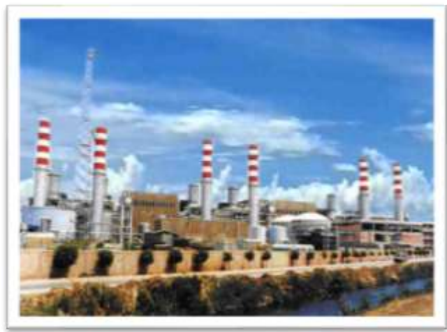
Damietta Combined Cycle Power Station
