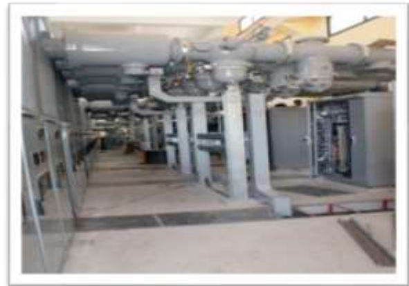
220 kV GIS Equipment
