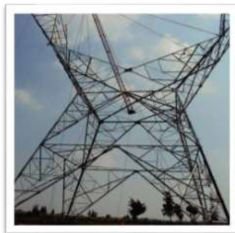
500 kV Single Circuit Tower
