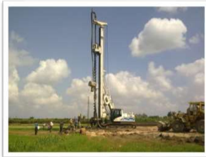
Deep Foundations (Piles) for OHTL
